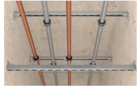
Pipe fixing in a corridor
