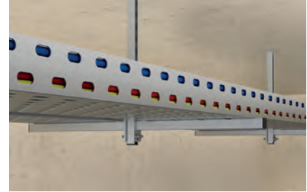
Suspended cable tray fixing
