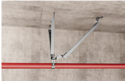
Pipe installation with seismic pipe clamp
