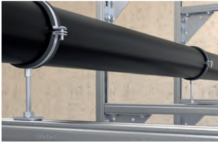
Connection on channel
