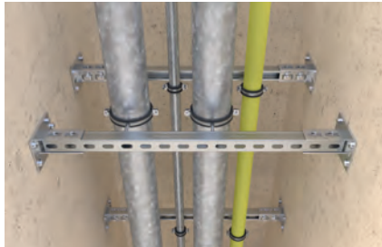
Pipe installation in escape route
