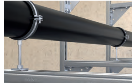
Connection on channel
