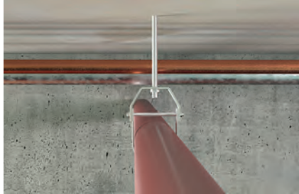
Sprinkler pipe installation
