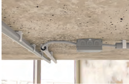
Fixing plastic insulating conduits
