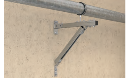
Upright pipe on cantilever arm
