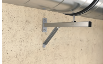
Ventilating pipe fixing at the wall
