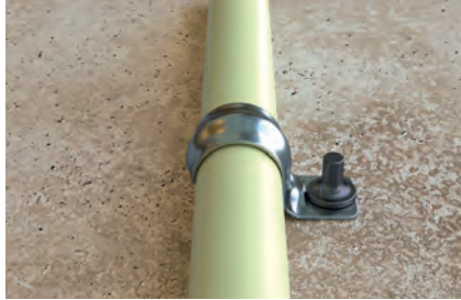
Fixing armoured conduits
