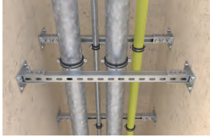
Pipe installation in escape route
