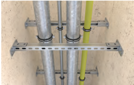
Pipe installation in escape route
