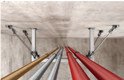
Bracing of frame construction with threaded rods
