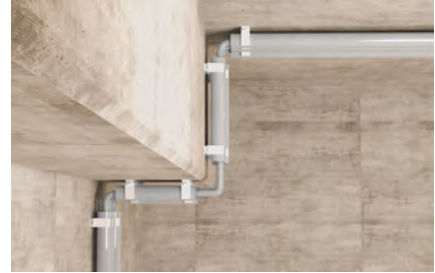
Fixing plastic insulating conduits
