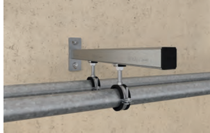
Light pipe fixing
