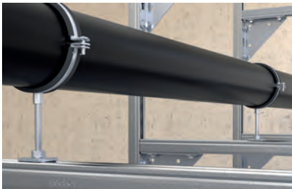
Connection on channel
