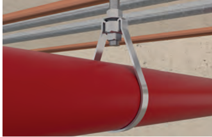
Sprinkler pipe installation
