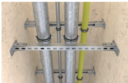
Pipe installation in escape route
