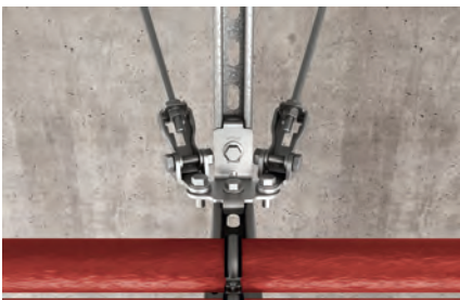
Connection of channel profiles and bracing elements
