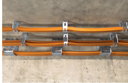
Cable fixing to the ceiling
