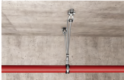
Bracing of pipeline with threaded rods
