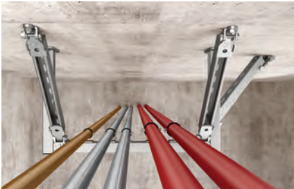
Bracing of frame construction with channel profiles
