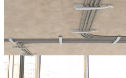
Fixing cable harnesses
