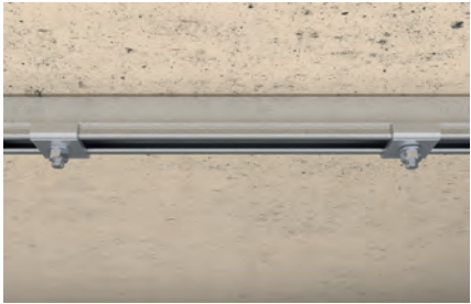
Channel installation at wall
