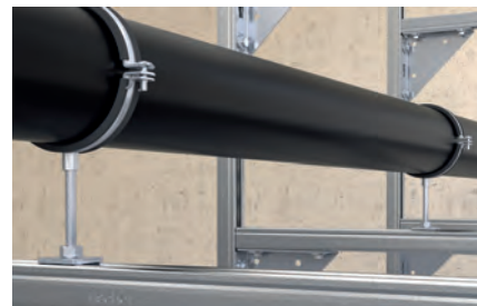
Connection on channel
