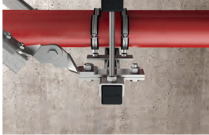
Bracing of channel construction
