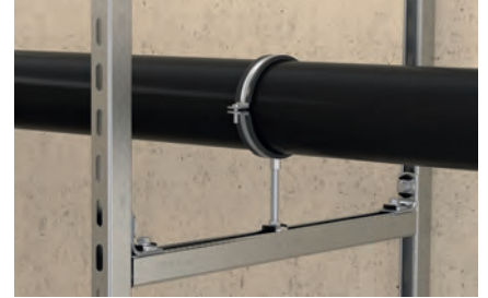
Pipe fixing on frame construction
