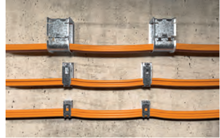
Cable fixing to the wall
